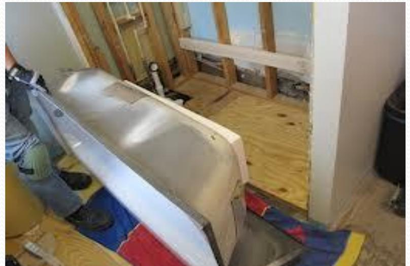
4.) Last, a pressed steel, polymer or fiberglass tub is then cut up into pieces for disposal. A cast iron tub can be covered with a tarp and smashed to bits.
