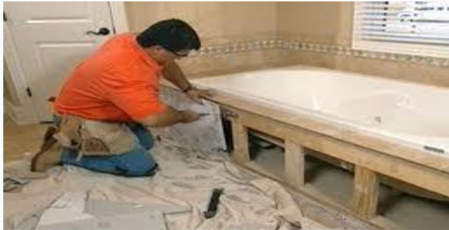
1.) First all plumbing fixtures are disconnected. Using a saw, at least 6 inches of wall is removed from around the tub. Now this looks like a simple process and can be depending what is behind the tile. If there is metal mesh and plaster which was typically used in the 60s then it is much more difficult. Also, consider the fact that matching that old tile is unlikely but not impossible, there are a couple of tile companies out there that re-manufacture the old look.
