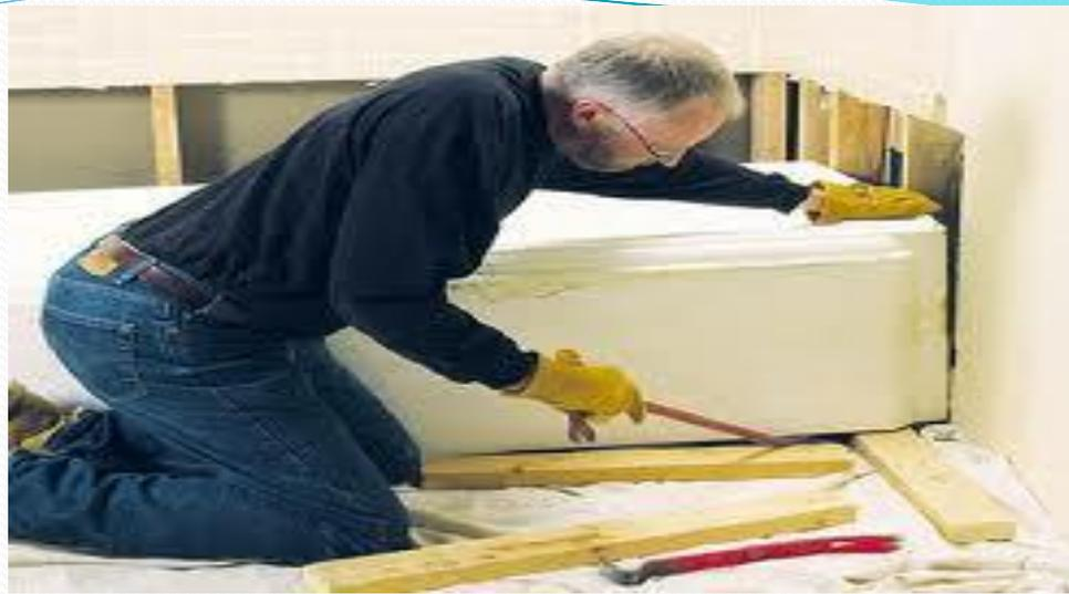
3.) Then the tub is lifted with a wrecking bar while soaped 1x4 wood skids are slid underneath. Now the tub will slide away on the skids. Sounds simple so far?
